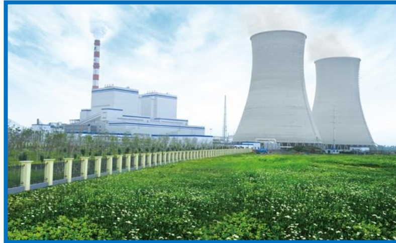
Circulating water situation
